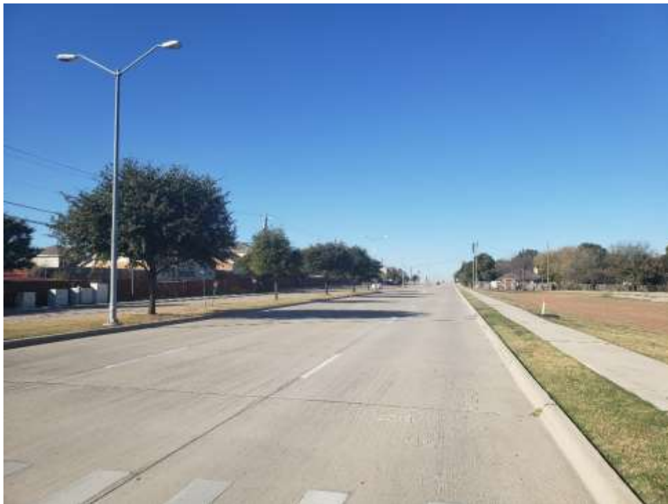
Street view of Longhorn Road looking west
