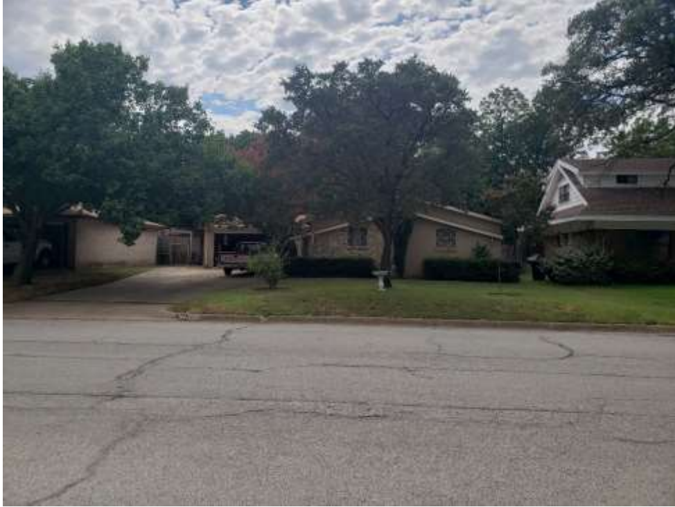
1. View of whole property from Opal street looking west.
