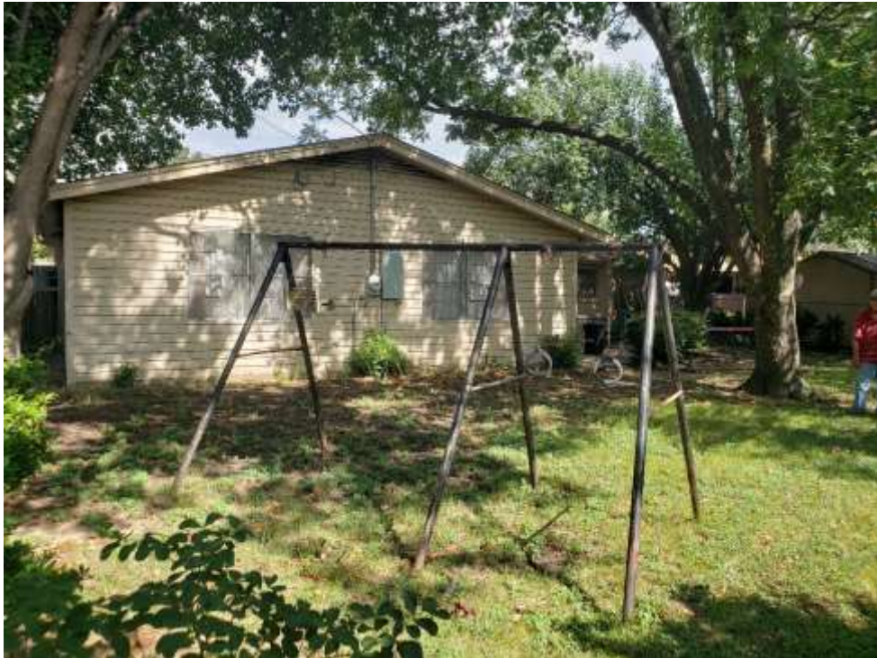
2. Rear view of property looking southeast from existing easement.
